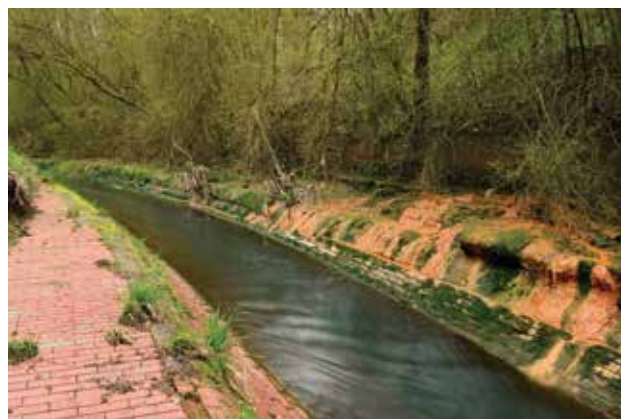
Figure 3.2 (Left) The Flesk River, Armoyle, a straightened channel in Northern Ireland (© Gareth Greer, Rivers Agency, Northern Ireland) and (Right) a section of the River Medlock in Manchester, England, a Victorian era brick-lined channel with a uniform shape before it was restored in 2014 (© RRC).
