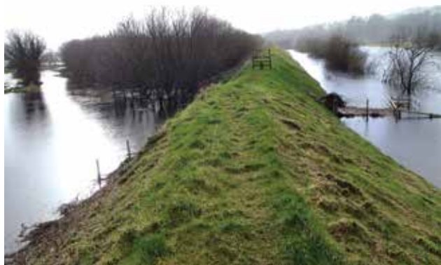
Figure 3.5 A flood embankment next to the Finn River, Clady in Northern Ireland. Flood defences prevent the natural exchange of water and material between a river and its floodplain (© Gareth Greer, Rivers Agency, Northern Ireland).
