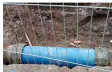
Image 13: Repaired pipeline after the major burst in Leicester 2015. (Source: DMU, 2015)
