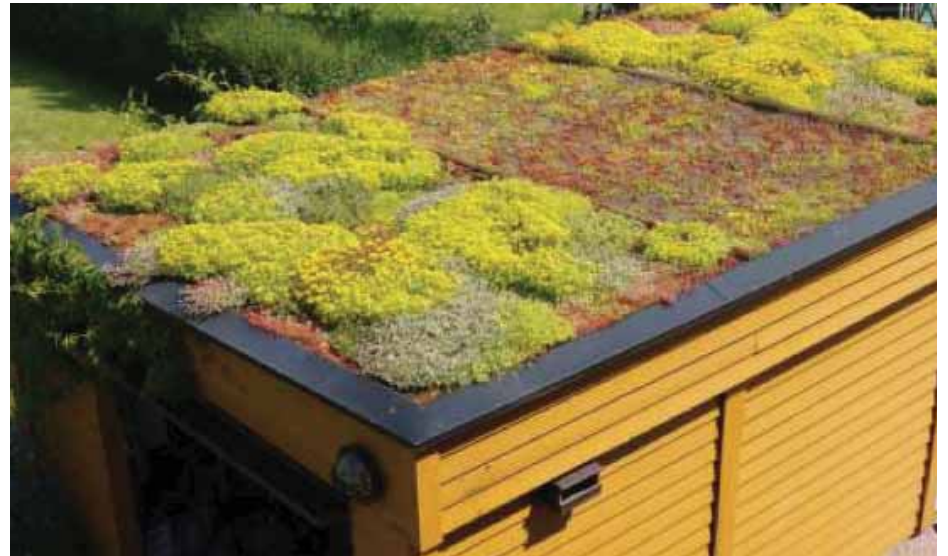
Image 7: Green roofs (Source: Braskerub et al., 2015)
